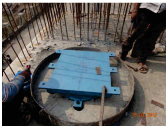
Photo 89 Rotating top plate after cutting Lock Clamp
