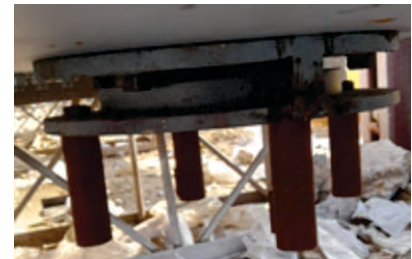
Photo 85 Bearing fixed with girder
