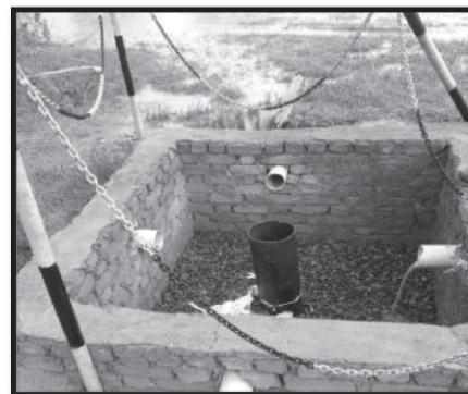
Rain water harvesting pit
