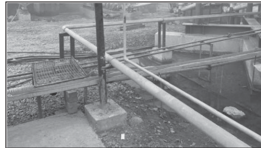
Piped Natural Gas used in Hot Mix Plant
