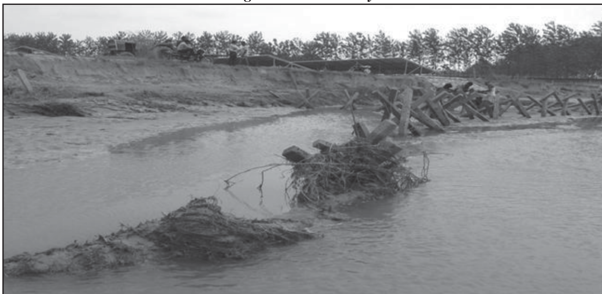
Fig. 2. Trapping of small trees and debris in Solani River, Uttarakhand, India by RCC Jack- Jetty
