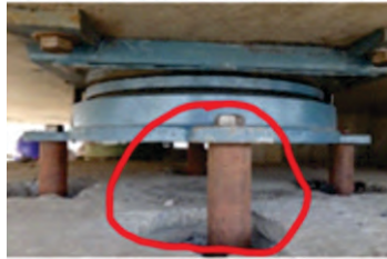
Photo-80 Low Pedestal height Photo 81 No proper assembling Photo 82 No proper assembling
