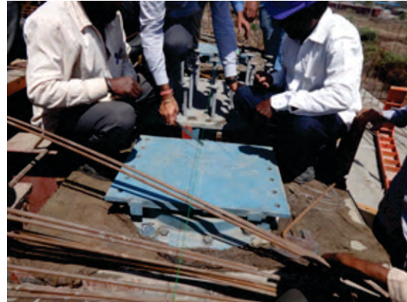
Photo 87 Rotating top plate after cutting Lock Clamp
