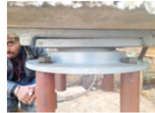
Photo-80 Low Pedestal height Photo 81 No proper assembling Photo 82 No proper assembling
