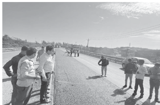
Photo: 3.3 Application of Terasurfacing on bituminous Pavement
