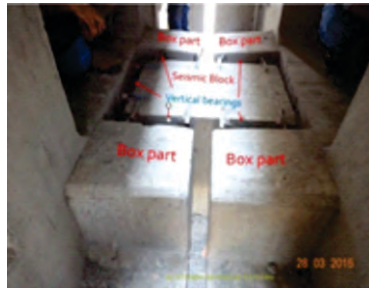
Photo-91, Sismic Block and Bearing
