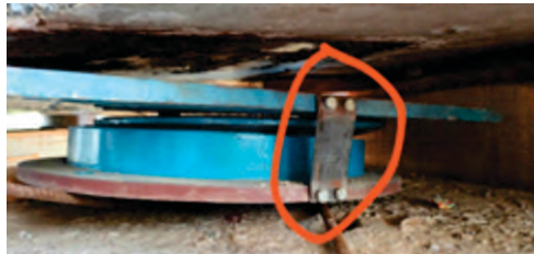
Photo-80 Low Pedestal height Photo 81 No proper assembling Photo 82 No proper assembling
