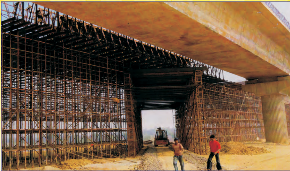
Flyover under RITES for DVC Project, Koderma
