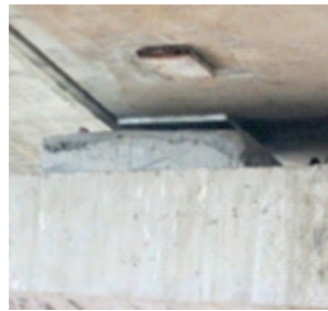
Photo-72 Steel Down stand
