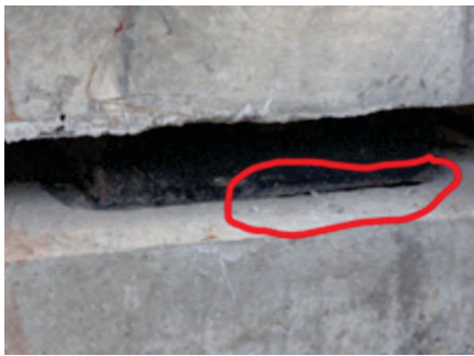
Photo- 67 Gap at bottom of Bearing
