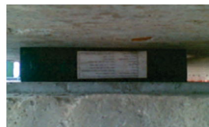
Photo 25 & 26 Elastomeric bearing fixed in position and loaded.
