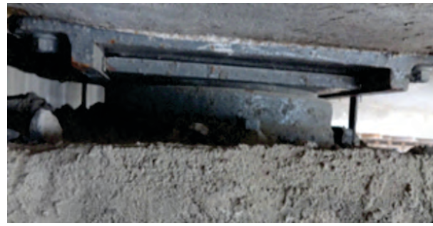
Photo – 59 Guided bearing in position
