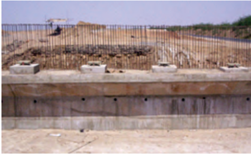
Photo 58 Pot bearings fixed for I-girders
