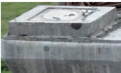
Photo-24 Recess for bearing
