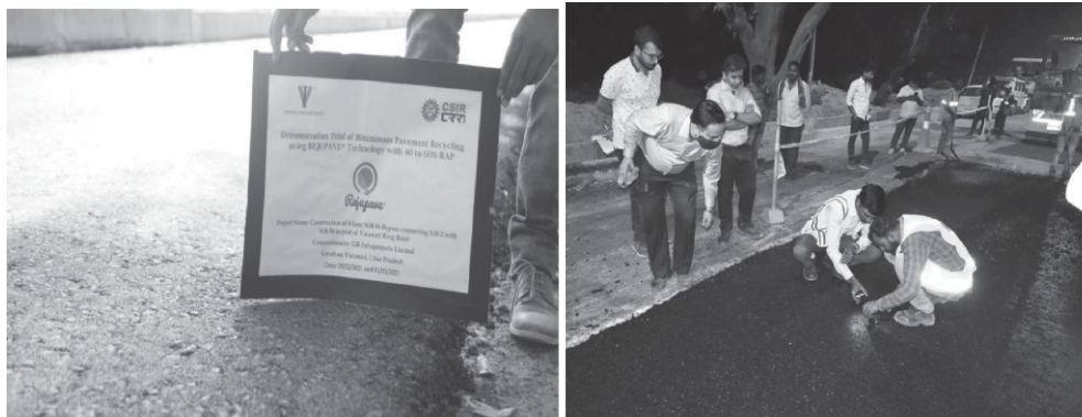
Photo 2.4: Glimpse of Test section constructed with 50 % RAP content in binder course layer
