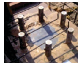
Photo 57 Bearing fixed
