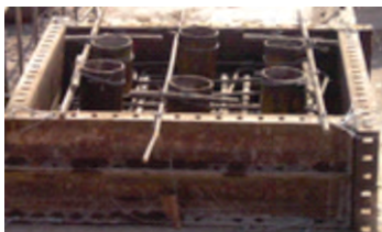
Photo 54 Sleeve hole position
