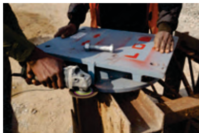
Photo 84 Lock Clamp cutting
