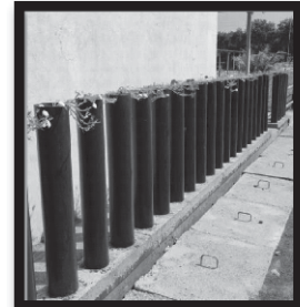
Waste Concrete converted to drain cover & scrap material used for beautification of site
