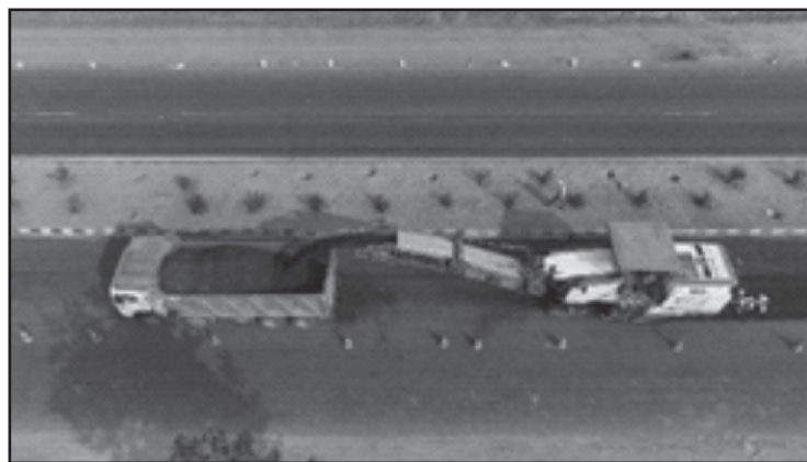
Milling of Existing Pavement
