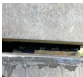
Photo 25 & 26 Elastomeric bearing fixed in position and loaded.
