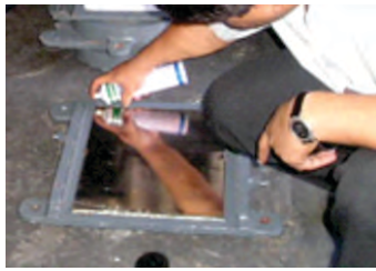
Photo-43 Cleaning of weld
