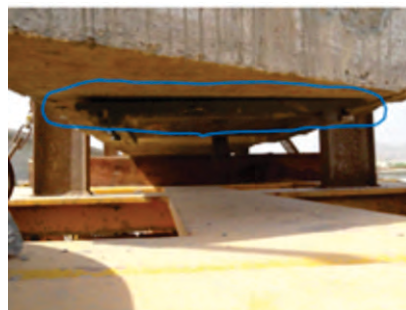
Photo- 78 Gap with girder
